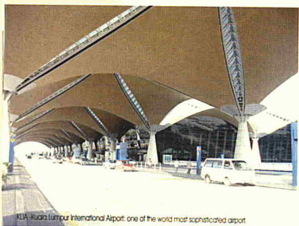
KLIA-Kuala Lumpur International Airport: one of the world most sophisticated airport
