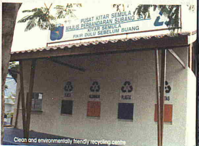
Clean and environmentally friendly recycling centre
