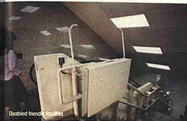
Disabled friendly facilities
