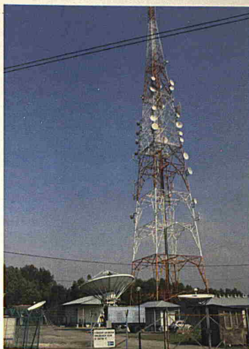
Satellite and telecommunication infrastructure
