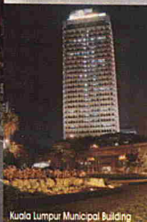
Kuala Lumpur Municipal Building
